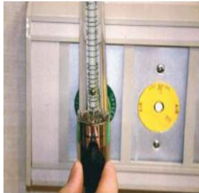
Figure 5. Flow Meter to Adjust Oxygen Flow
