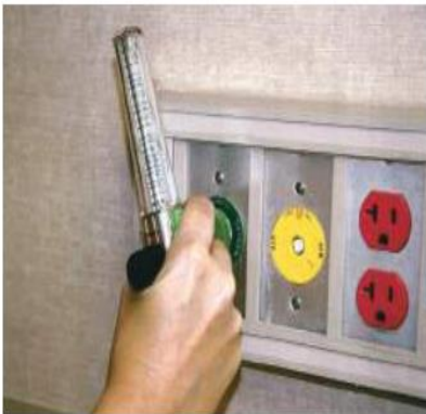
Figure 5. Flow Meter to Adjust Oxygen Flow
