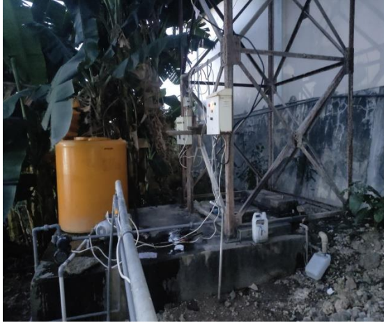
Reservoir Asrama Kebidana Poltekkes Kemenkes Kupang
